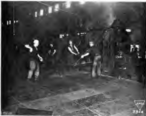
ROLLING IRON INTO SHEETS
